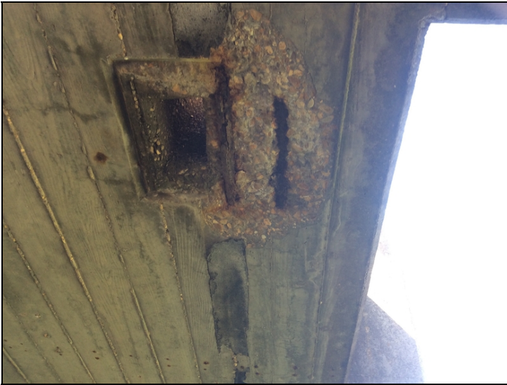
Delams with exposed steel around drains
