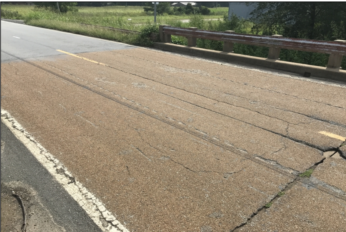
Wearing surface - Span 3: Cracking
