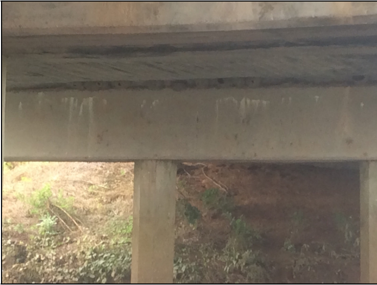
Large cracks with efflorescence on bent 2 cap ahead.
