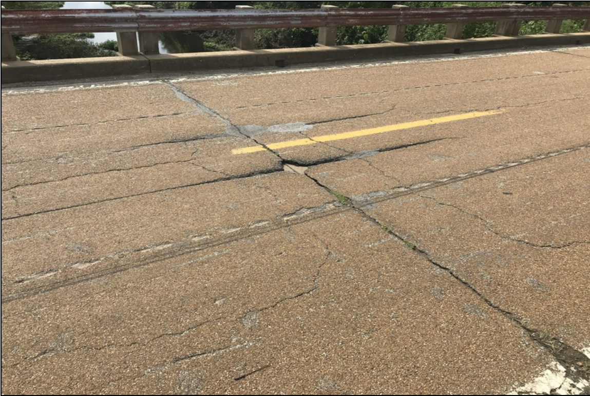
Wearing surface @ Bent 3: Cracking/spalling
