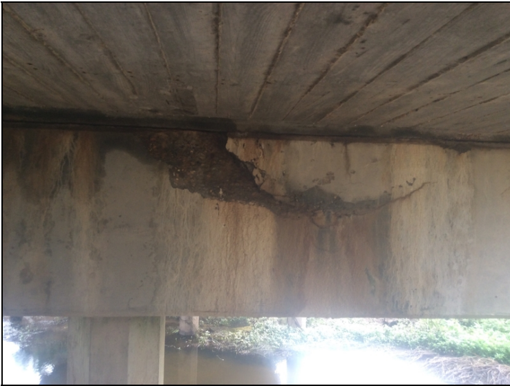
Bent 2 back near mid span has delam.
