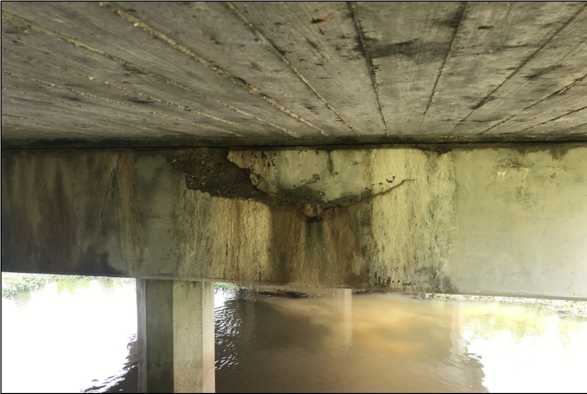
Cap - Bent 2 back right: Spalling/delamination
