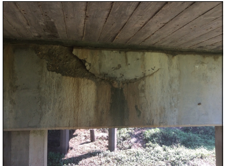
Large Delam on bent 2 cap .
