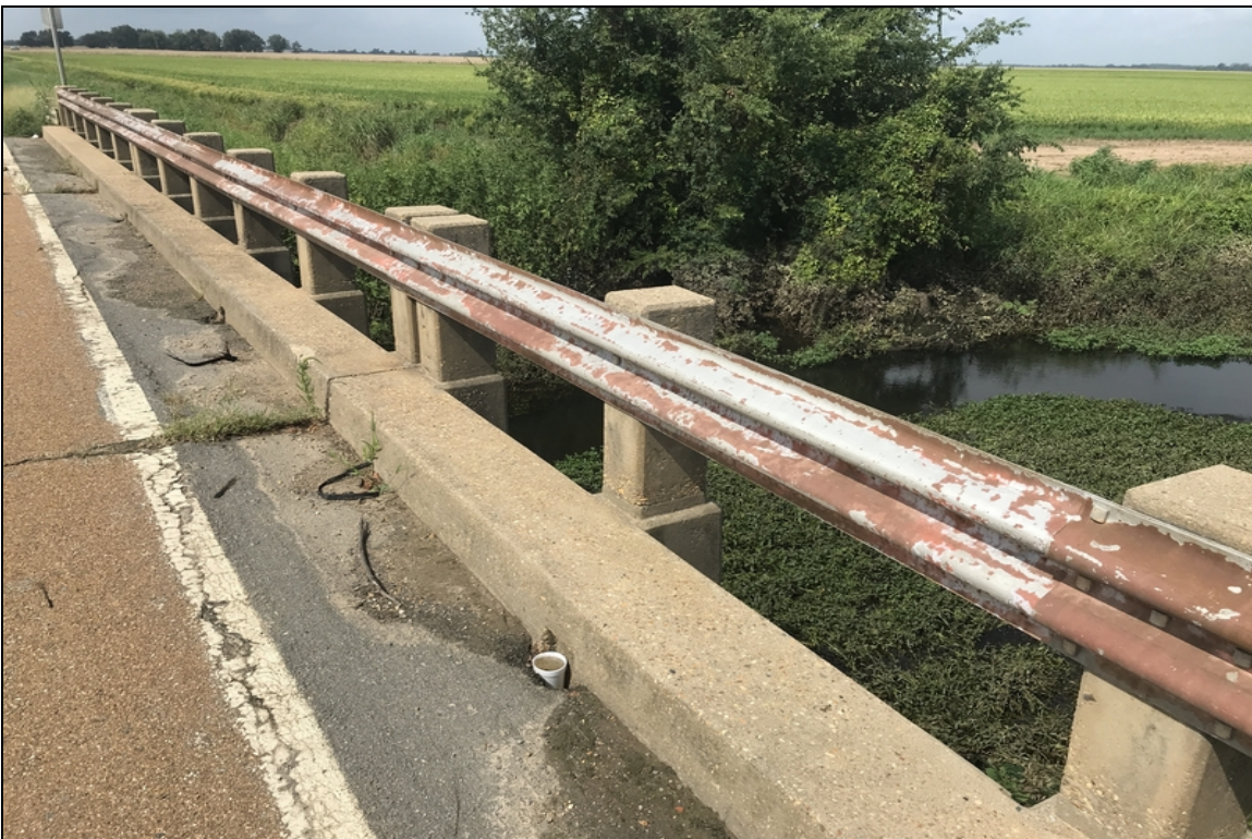
Railing - Spans 2-3 left: Paint peeling
