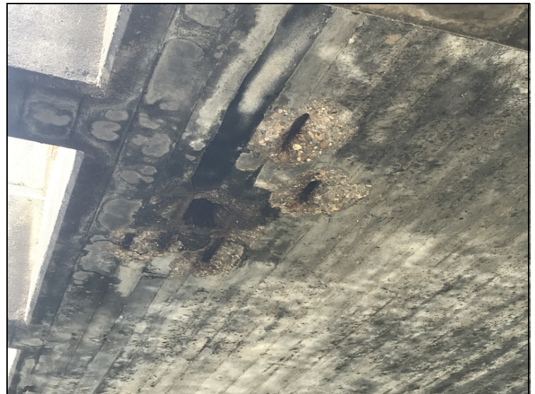
Soffit - Span 2 right: Exposed Rebar @ drain
