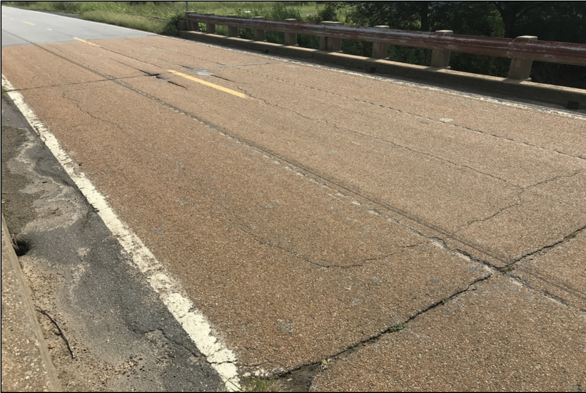
Wearing surface - Span 2: Cracking
