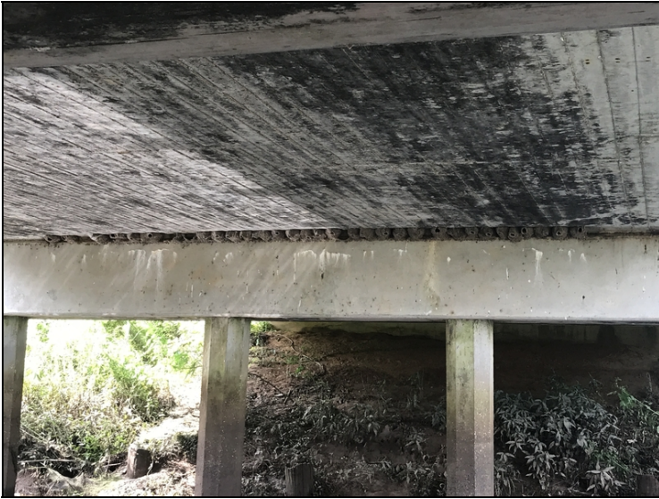
Cap - Bent 2 ahead: Efflorescence
