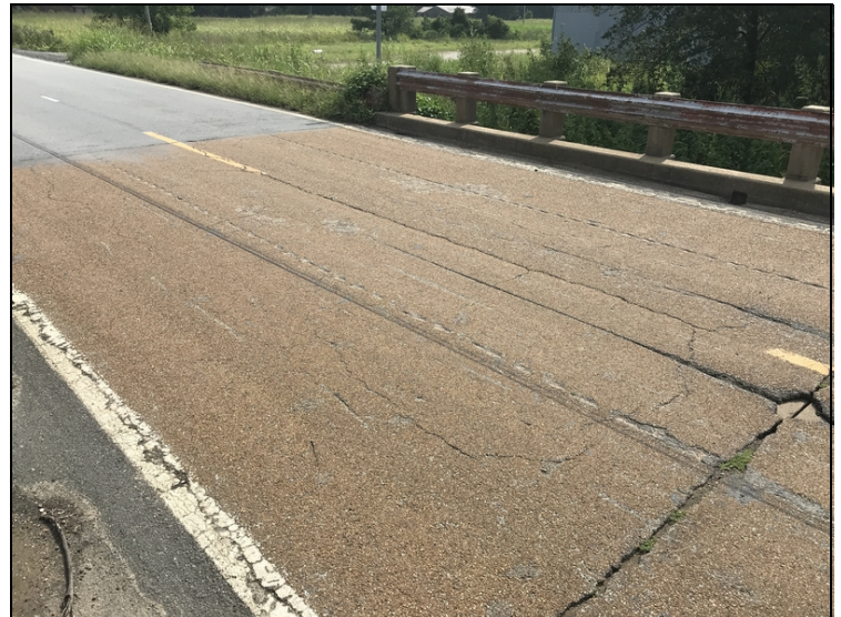
Wearing surface - Span 3: Cracking
