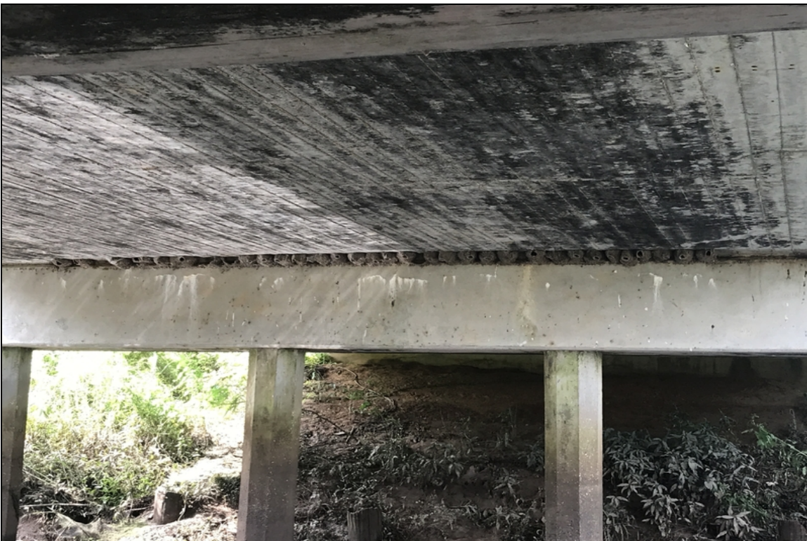
Cap - Bent 2 ahead: Efflorescence
