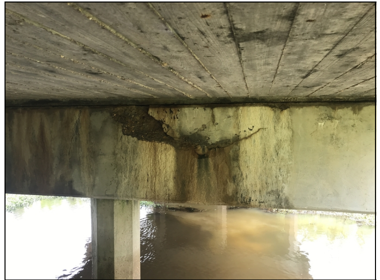
Cap - Bent 2 back right: Spalling/delamination
