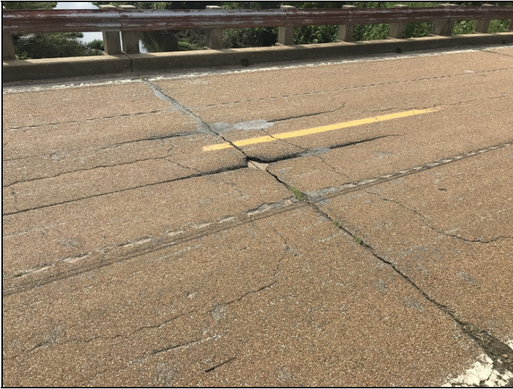
Wearing surface @ Bent 3: Cracking/spalling
