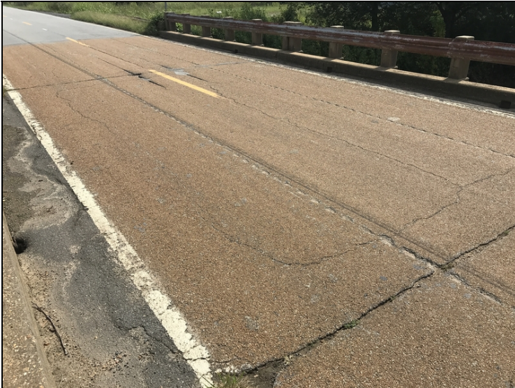
Wearing surface - Span 2: Cracking
