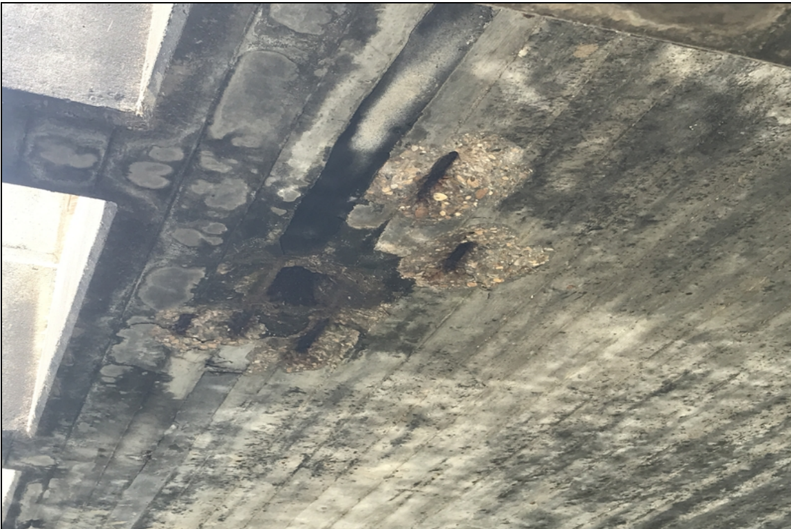
Soffit - Span 2 right: Exposed Rebar @ drain
